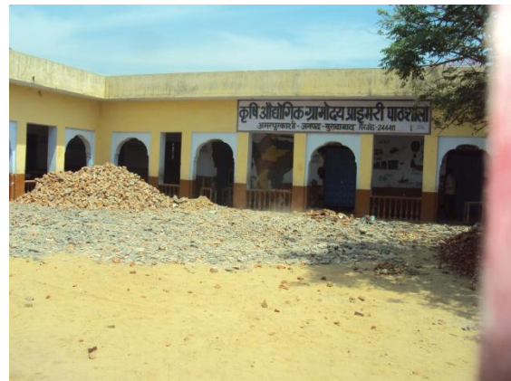
Work in progress to resurface the playground of the primary school
