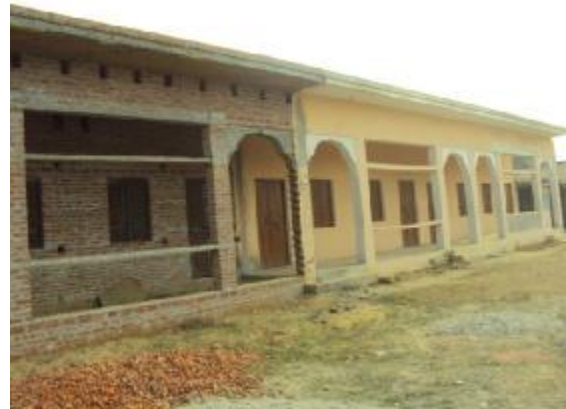
Two completed classrooms at Jafarpur High School and one in progress
